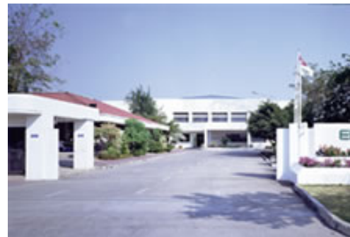
Factory in Thailand
